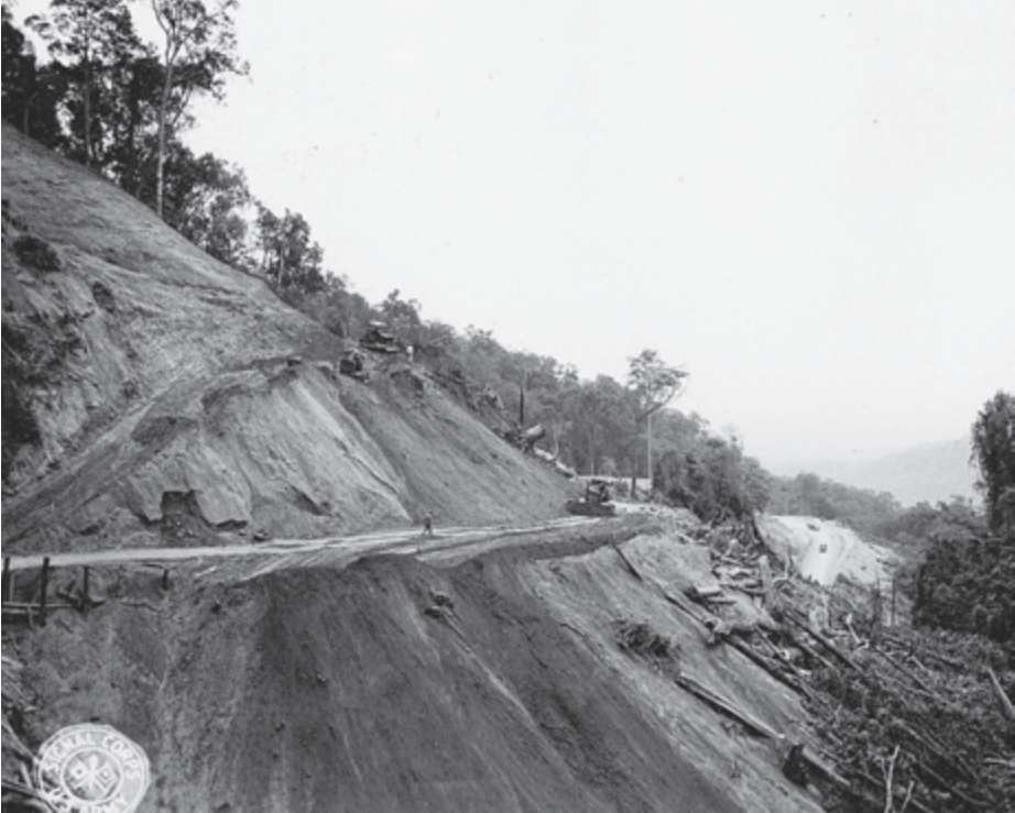
Along the Ledo Road, April 28, 1945. Bulldozers are shown making a new cut at the 96-mile mark on the Stilwell Road in Burma (National Archives: 111- SC-273003).
